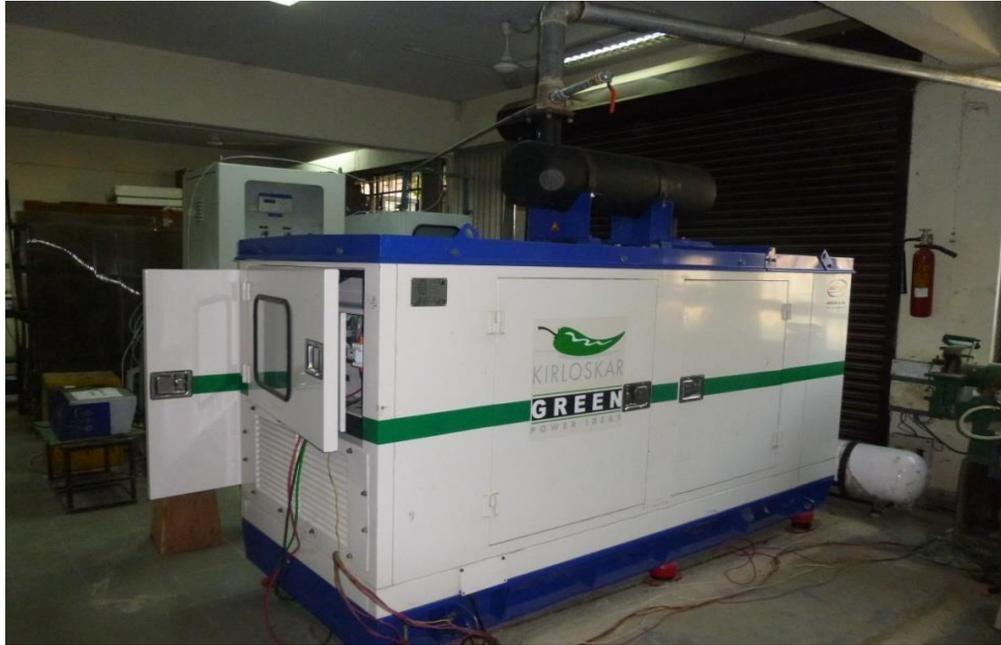
Figure 14: A photographic view of a hydrogen-fuelled generator developed in IIT Delhi with MNRE funds/support.
